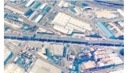
The collapsed section of the Nimitz Freeway.
