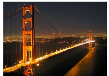
w / The Golden Gate Bridge's roadway is held up by the tension in the vertical cables.
