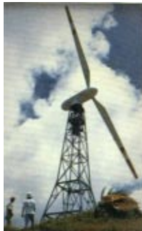
Figure 1: Truss tower supporting the NASA wind turbine generator at Oahu, Hawaii.
