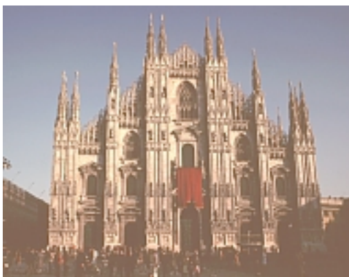
The main Entrance Portal
